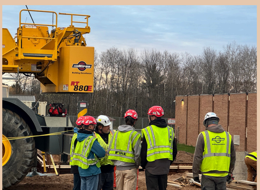
In November, the MASH Highway Construction Skills students traded their morning lesson for a hands-on experience with Miron Construction, the general contractor for the district's referendum-funded projects. These students arrive at 7 a.m. each day, before regular classes, to earn their certification toward becoming skilled heavy equipment operators.
