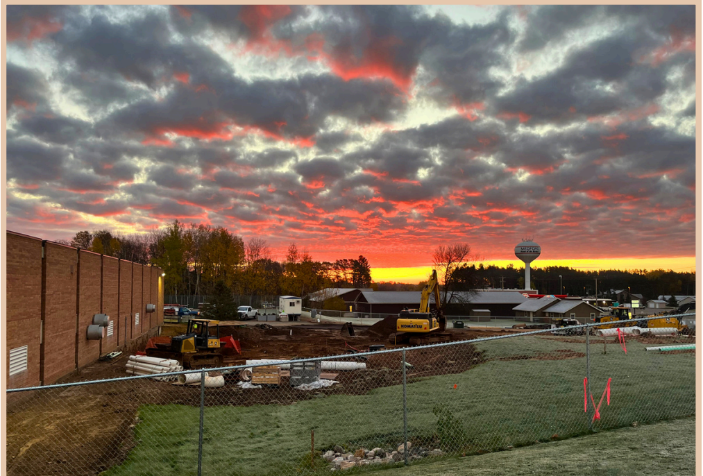
The late October sun rises over MASH's south construction site, where crews are building eight new classrooms for science, art, and family and consumer sciences.
